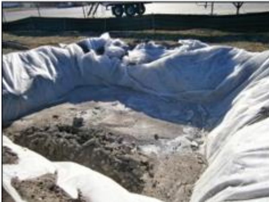
Plate 4-4 Concrete Washout Area
