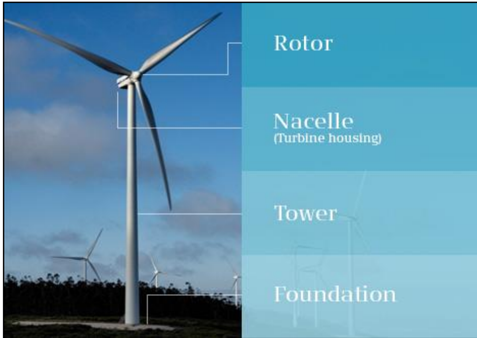
Plate 4-1 Wind turbine components
