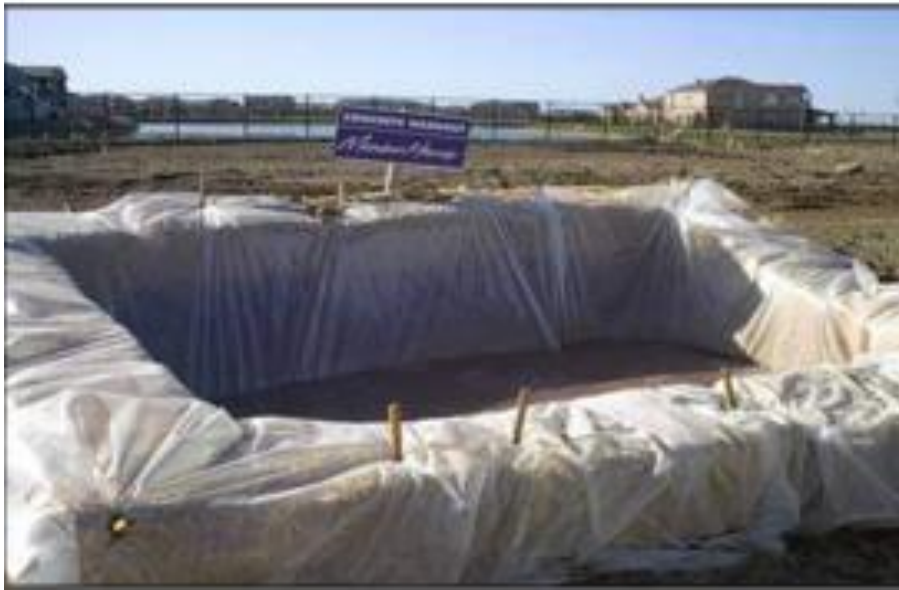
Plate 4-3 Concrete Washout Area
