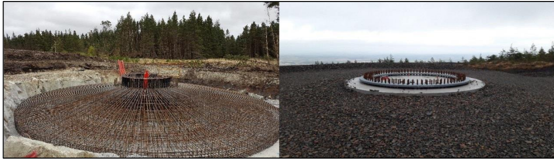
Plate 4-2 Turbine 'Anchor Cage' and finished turbine base
